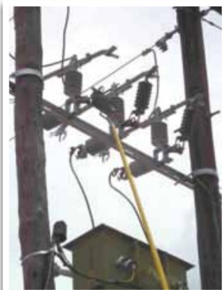
Fig.8 The live line surge arrester in the Combi unit is positioned not further than 1 meter from the transformer, Eskom specification, D-DT-1877.
