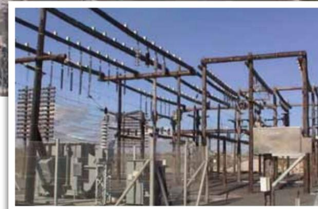
Fig.1: Koeberg Insulator Pollution Test Station (KIPTS).
