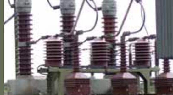
The accuracy must be within 0.25% for type X CT's and 0.2% for metering CT's. or it is rejected.
