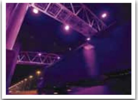
Figure 6. Lights used to illuminate the vehicle license plates.
