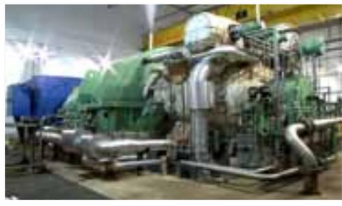
*A TGM condensing extraction steam turbo generator set operating at a paper mill in Brazil. This set is similar to that which will be supplied and installed at Mondi Richard's Bay facility.*
