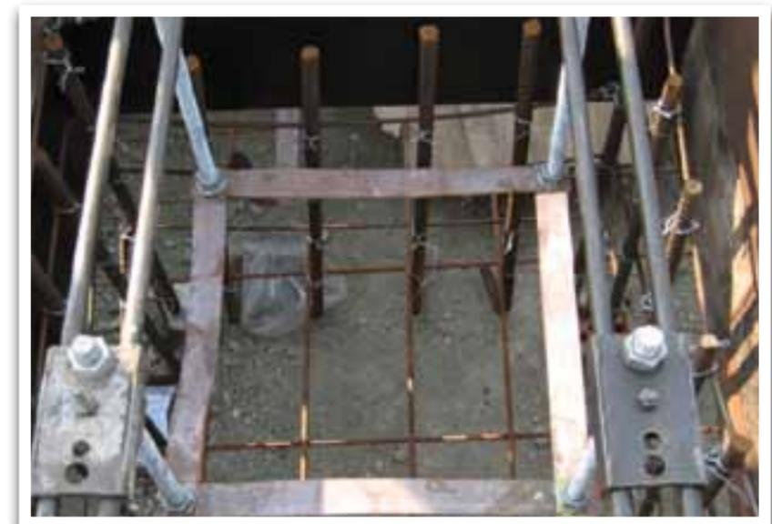
*Concealed copper earthing in foundation as applied in Eskom Distribution*
