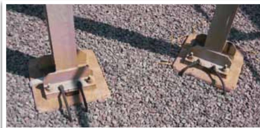
Copper plated steel earth rods used for the earthing of structures in Eskom Distribution
