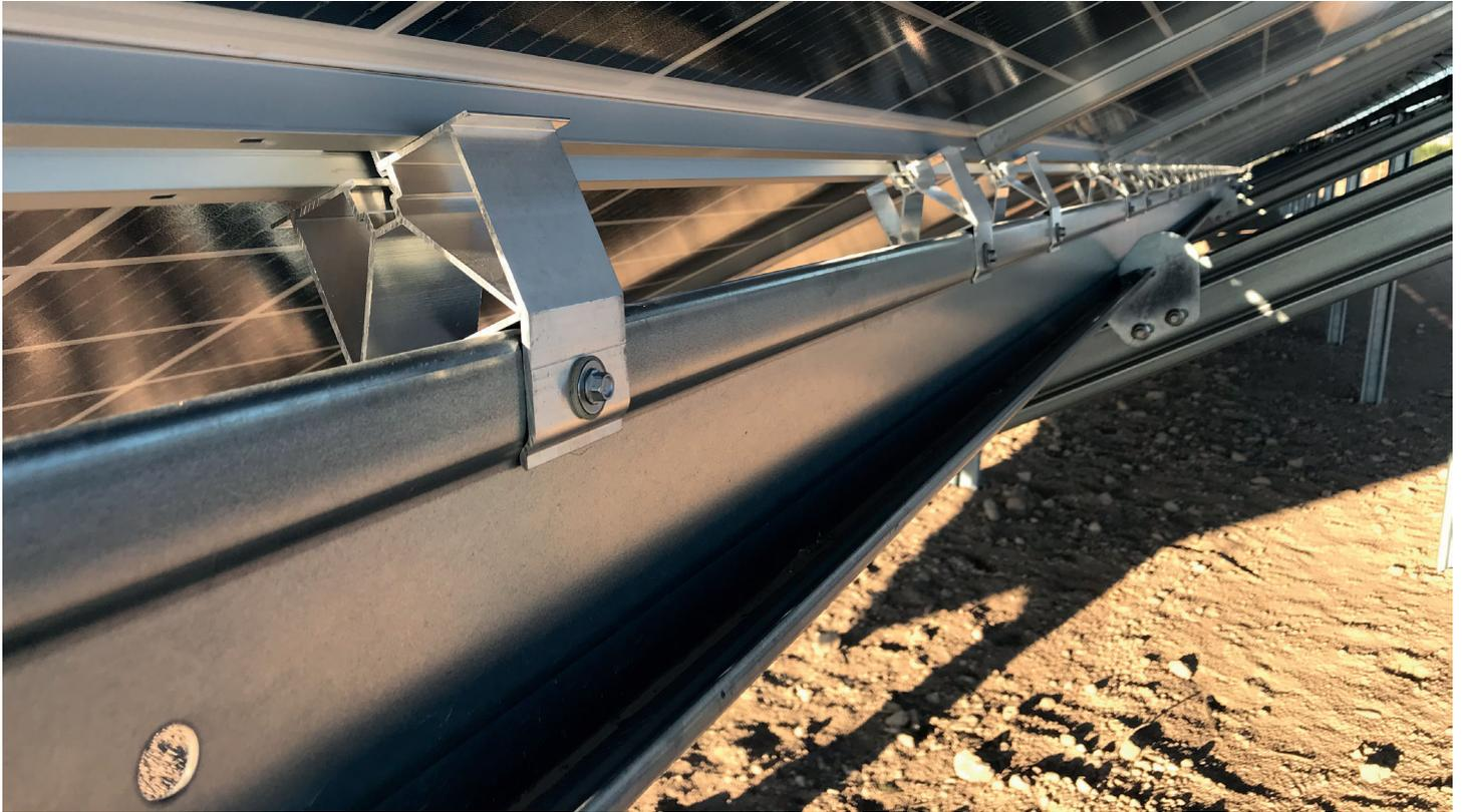
The trend towards bifacial modules continues: The Schletter Group has supplied the mounting systems in Spain for a 2 MW open area plant of Spanish project developer Atersol. To optimize the yield from the plant, Schletter developed a new module clamp adapter for the project. This reduces shading on the underside of the module considerably.
