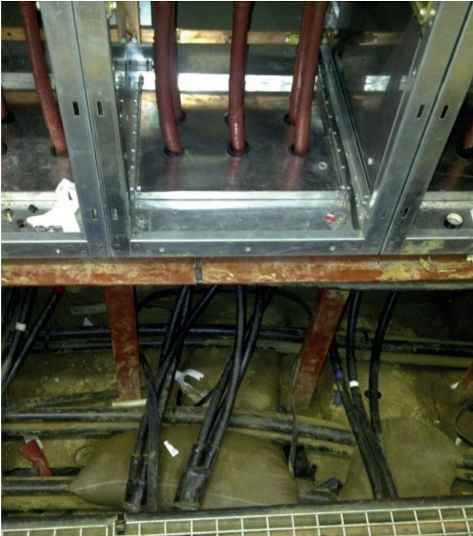
Picture 6: Example of tri-furcating termination into compact MV switchgear.
