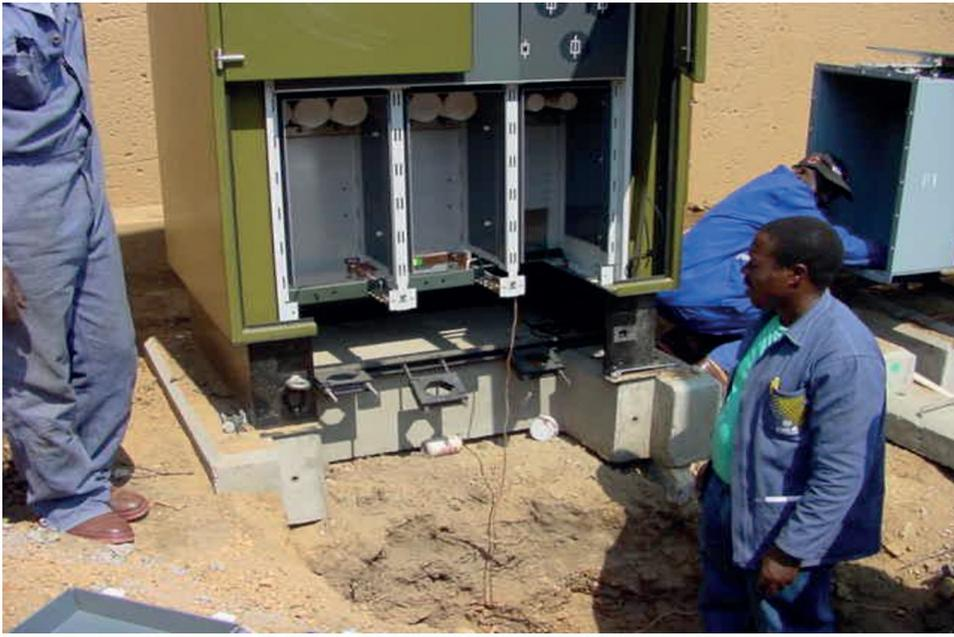
Picture 5: Example of SF6 RMU with an additional raising plinth and removable front sections.
