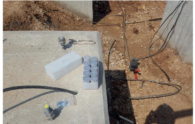
Examples of copper clad steel (CCS) being installed for substation earth grids in accordance with NRS 102.
