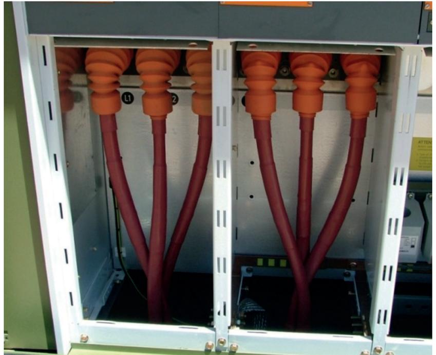
Figure 11: Example of a cable termination where the core crossing is made below the end of the core screen.
