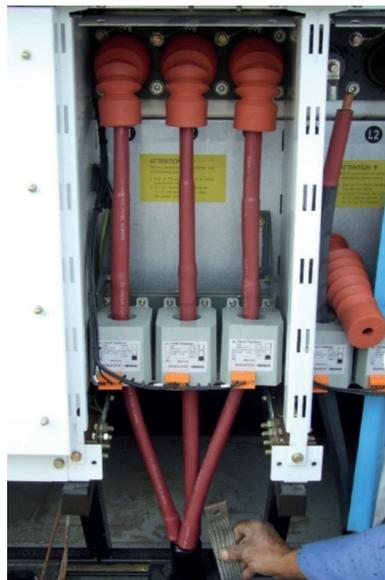
Figure 10: Illustration of the correct earthing for ring-type current transformers on each cable core used for overcurrent and earth fault detection.
