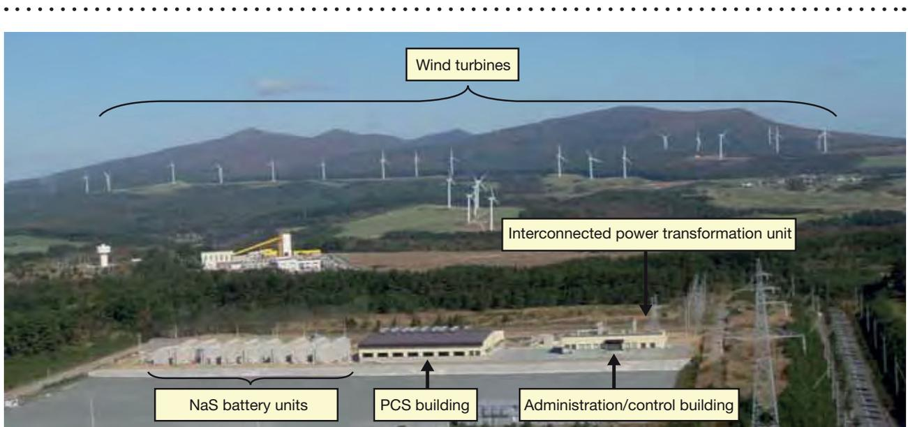
**Figure 3-9 | General view of the Futamata wind power plant** (*Japan Wind Development Co.*)
