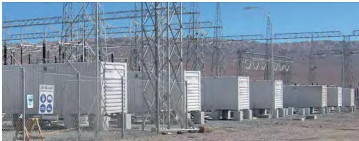
**Figure 3-3 | Li-ion battery supplying up to 12 MW of power at Los Andes substation in Chile**
