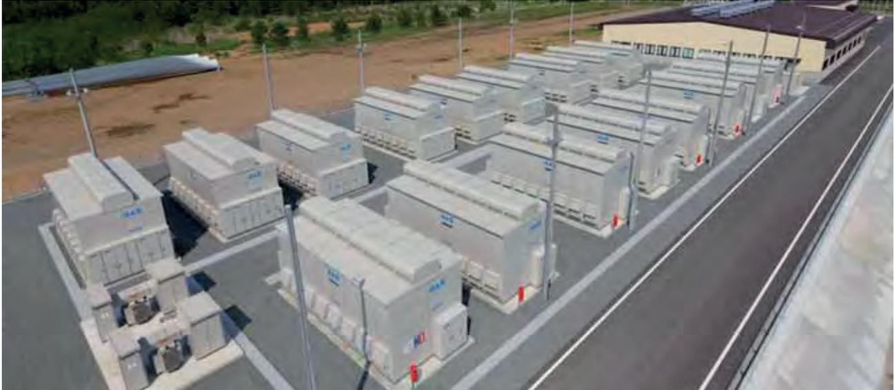
**Figure 3-10 | NaS battery units – 34 MW** (*Japan Wind Development Co.*)
