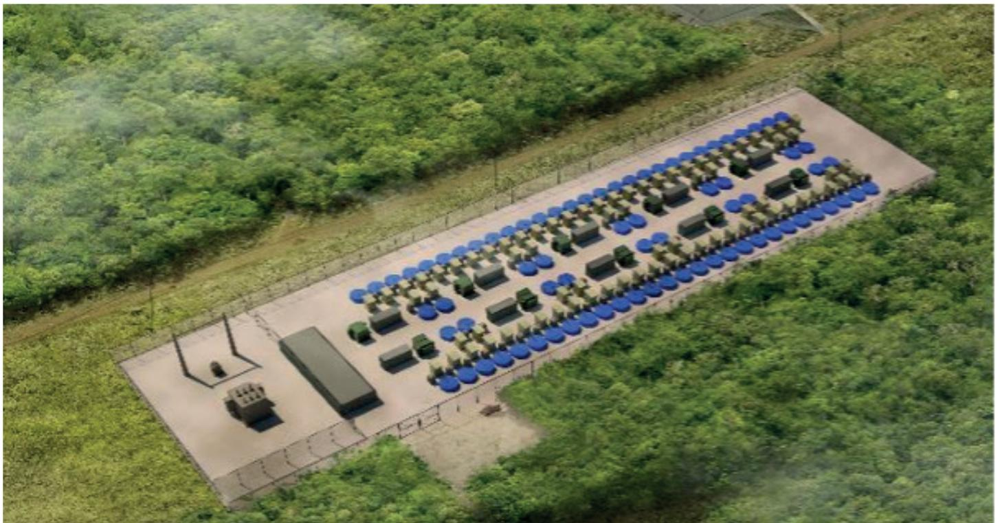
*Beacon Power 20 MW 5 MWh flywheel energy storage*
