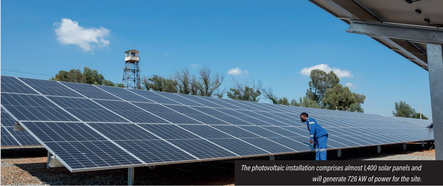
*The photovoltaic installation comprises almost 1,400 solar panels and will generate 726 kW of power for the site.*
