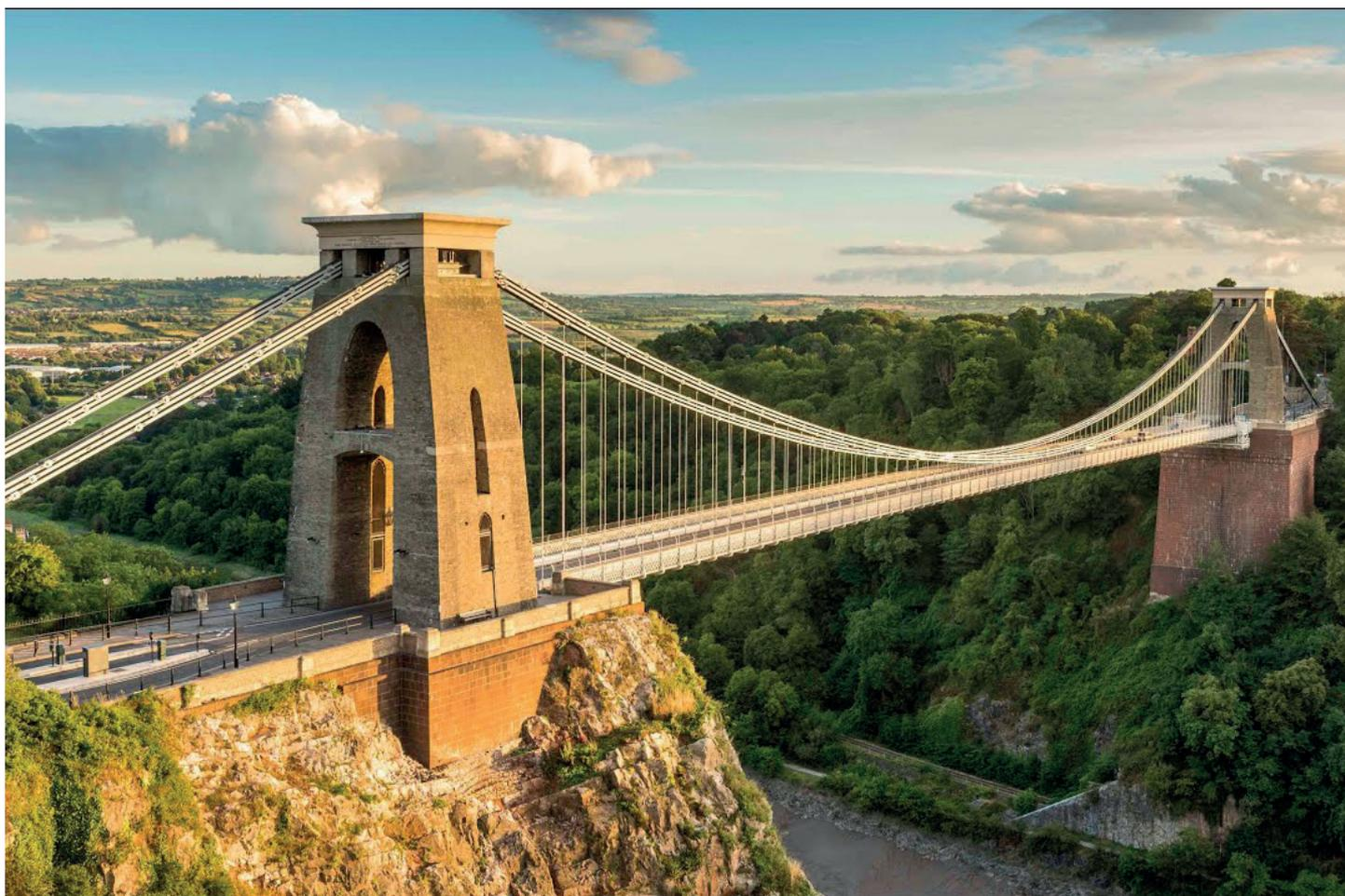
*I K Brunel's famous Clifton suspension bridge started in 1851. At this time, plate-chains were used for catenaries. Some of the chains were salvaged from the demolished London Hungerford Bridge over the Thames.*
