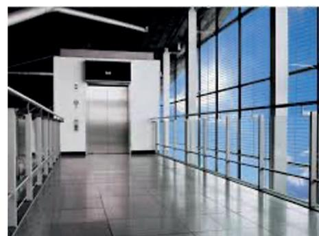
*Figure 3: The visible light is let through while ultraviolet and infrared rays are redirected to small solar panels on the side of the glass.*
