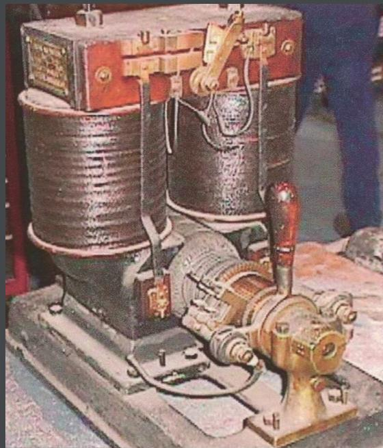
DC machine and the brush gear position had to be advanced or retarded by hand to suit the load conditions.
