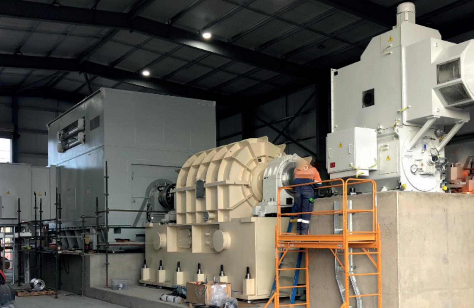
*Synchronous condenser being installed, showing synchronous condenser, flywheel and starting motor.*
