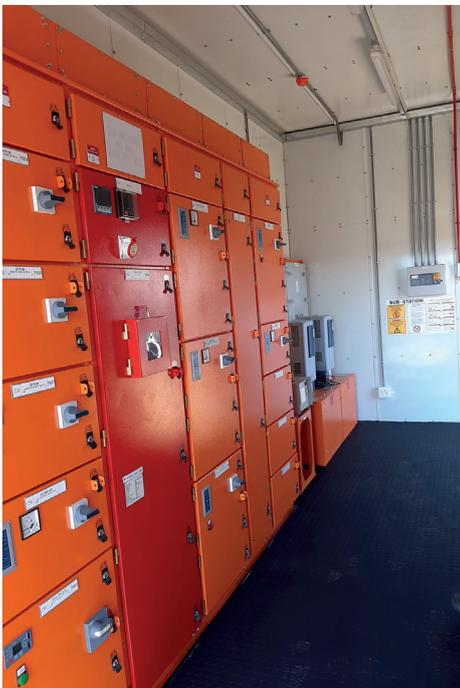
*The low voltage (LV) room of the E-House with the internally arc type-tested IEC 61641 MCC.*
