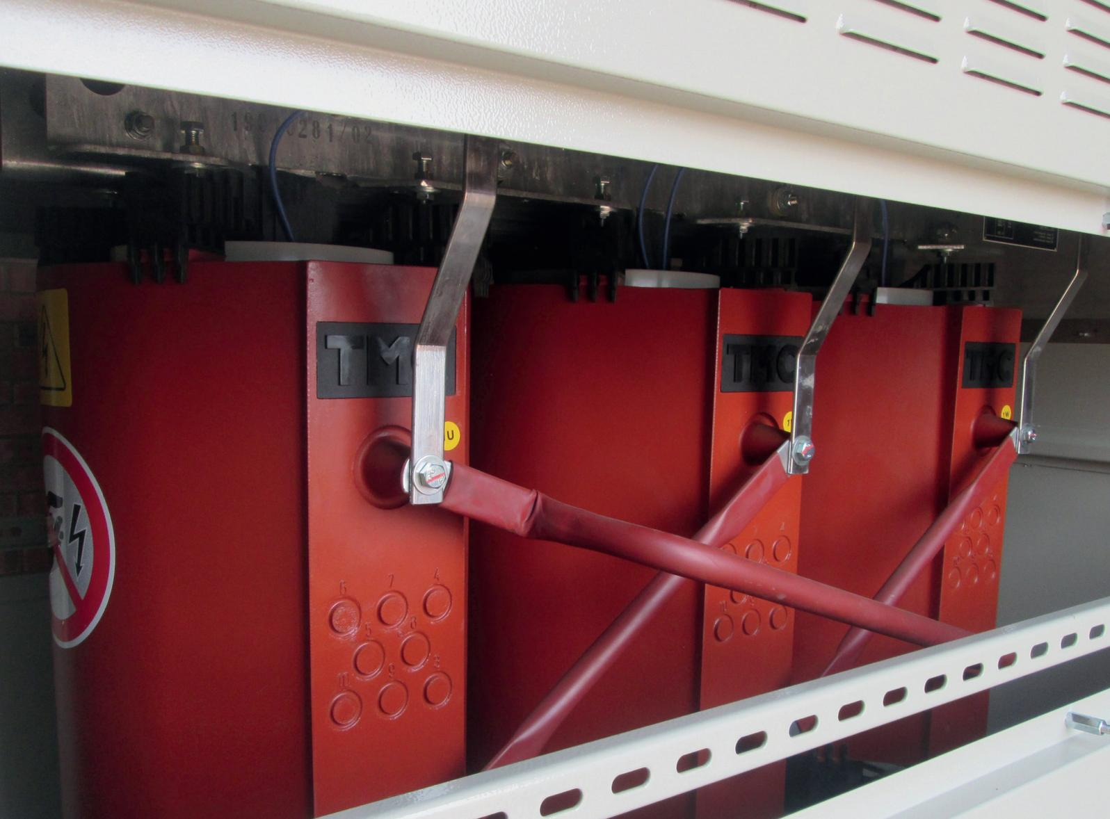
*A 400V/22kV step-up transformer designed for renewable energy applications.*
