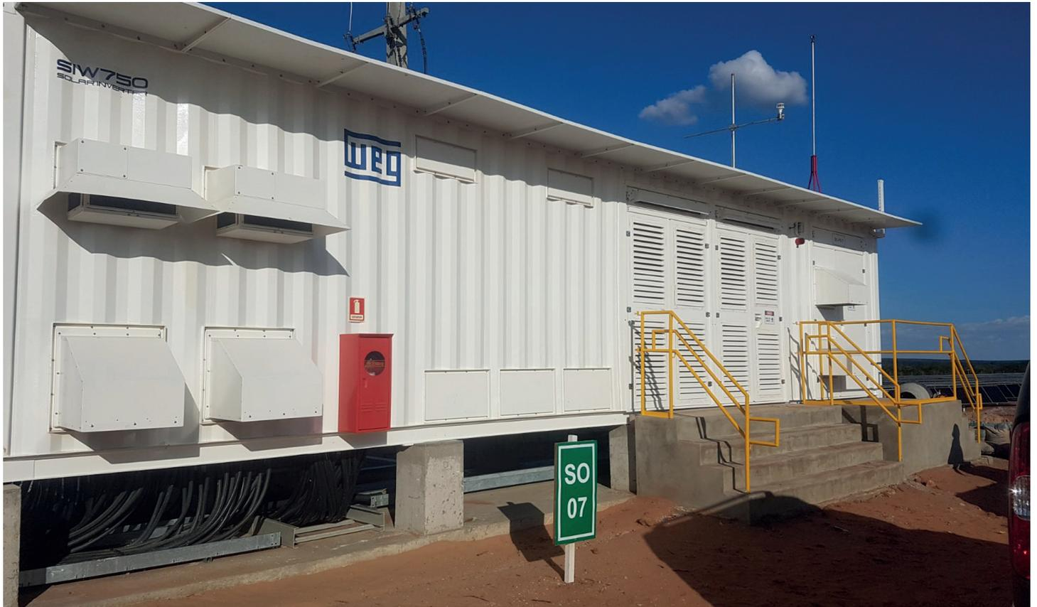
*The WEG ESW 750 centralised inverter station, housed in a 12 metre container installed on site.*
