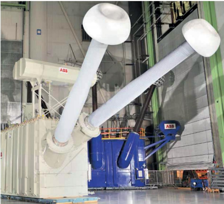
*ABB (ASEA Brown Boveri) UHV single phase converter transformer*
