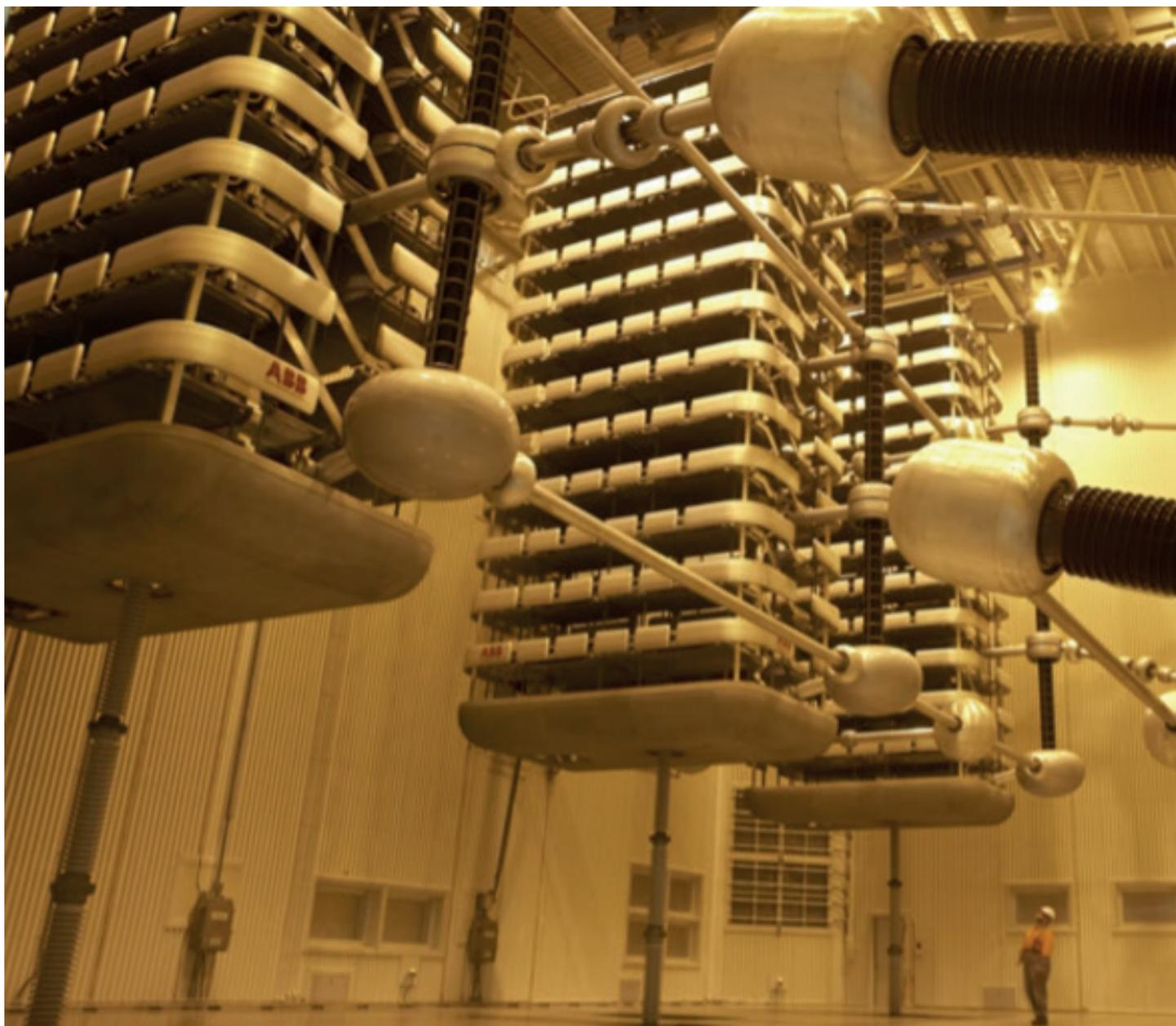
*Suspended twelve-pulse ABB thyristors in the valve hall at Haywards in the New Zealand HVDC Inter-Island scheme
