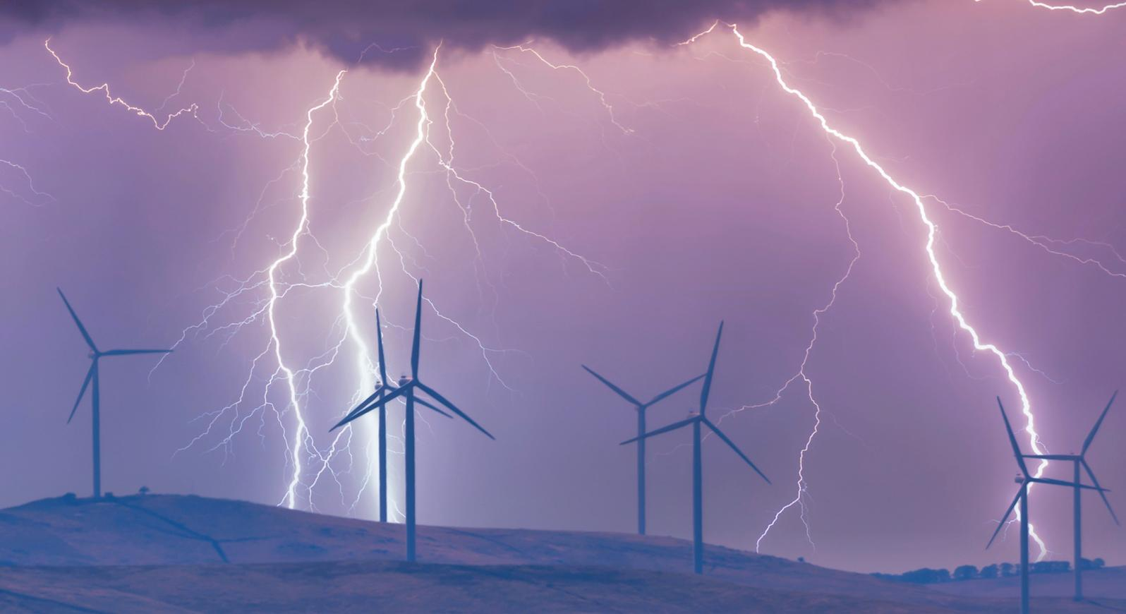
This is mainly due to the phenomenon that tall structures (especially Wind Turbines) are subjected to upward lightning more frequently than it would be to downward lightning. Downward lightning strokes, make up more than 90% of all recorded lightning strikes globally (IEC 62305-1), but upward lightning carries higher peak values of current and carries more charge content, causing more damage. The concept for upward lightning and downward lightning is shown in Figure 1.
