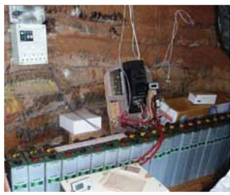
Fig 8. The regulator (black) regulates the voltage for the 24 batteries and the inverter, inverts the 48V DC to 220V AC.
