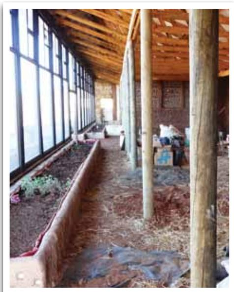
Fig 10. The two planters are on the left, inside the northern windows. At the back, see the wall made of bottles and cans. Earthbag walls are being plastered on the right.
