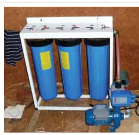
Fig 9. The water filter system.
