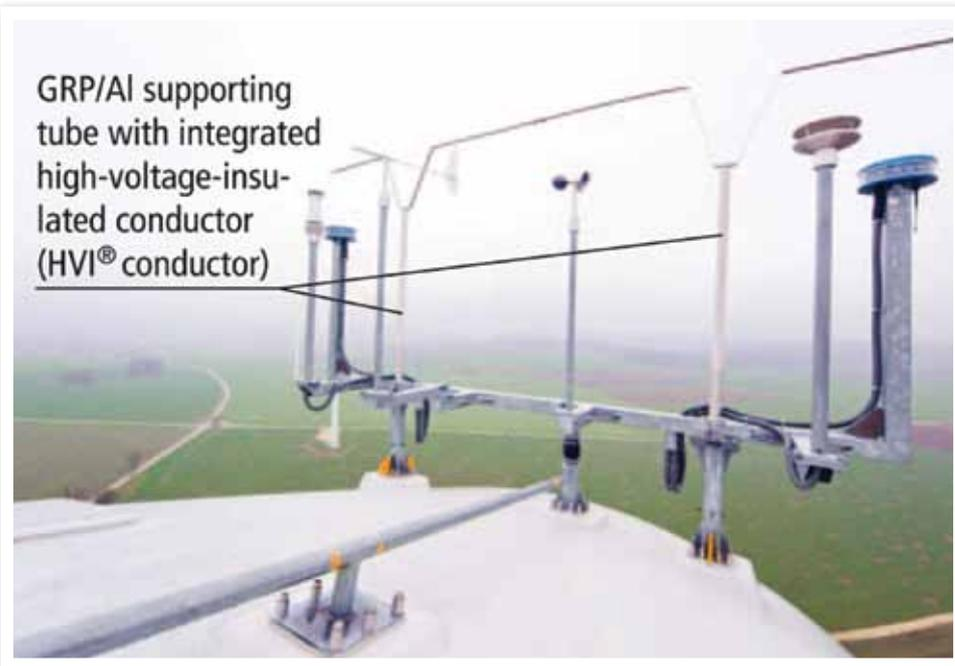
Figure 2 - Example of an air-termination system for the weather station (anemometer) and the aircraft warning light
