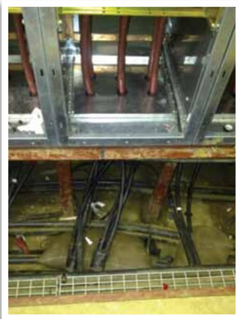
*Example of tri-furcating termination into compact MV switchgear*
