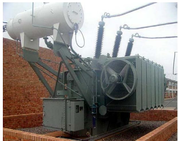
Fig. 9: Picture of 132/11 kV Transformer, 30 MVA
