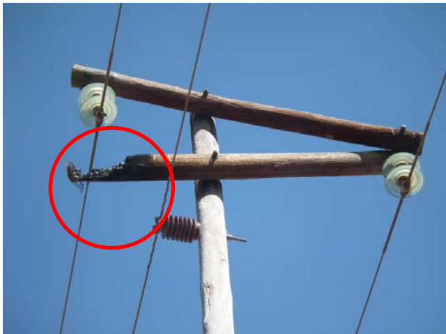
Figure 4: Wood pole cross-arm after a fire caused by leakage current flow
