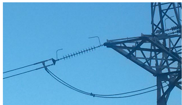
Figure 1: 132kV arcing horn arrangement
