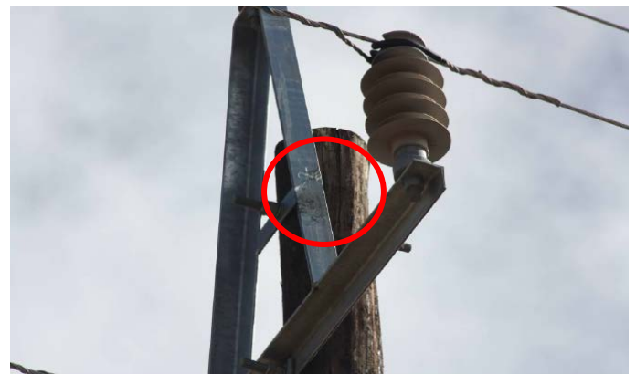
Figure 2: Burn mark on the metal frame of the intermediate structure after a martial eagle was electrocuted [3]
