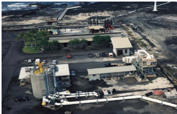
Fig 1: 210-Kilowatt Open-Cycle Ocean Thermal Energy Conversion Experimental Apparatus.
