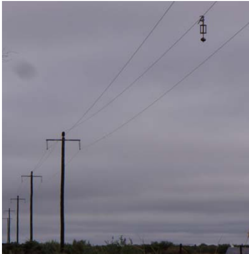
Fig 2: Spark-gap device mounted on the line at point SG2
