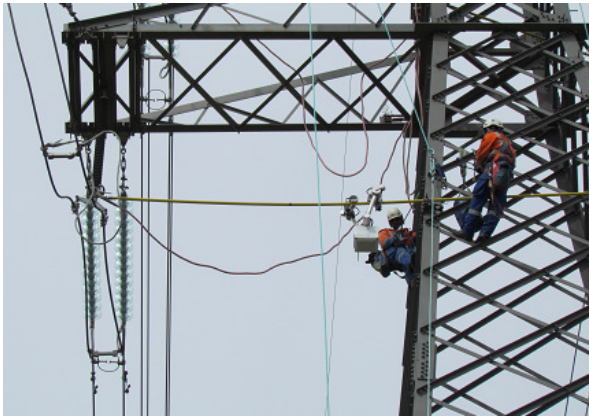
Figure 1: Insulated rod used as bridge for deployment
