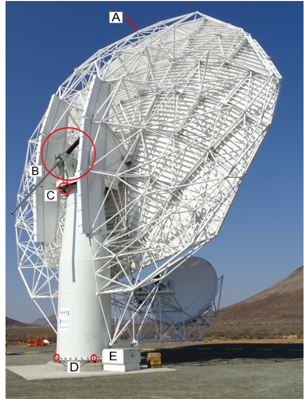
Figure 7: Earlier MeerKAT antenna photograph with circled points of interest: A: Current injection point, B: Jack screw assembly, C: Shoe-slipring assembly, D Pedestal-to-earth connections, E Isolation transformer.
