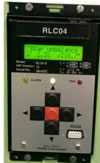
Figure 5: Current unbalance level on commissioning
