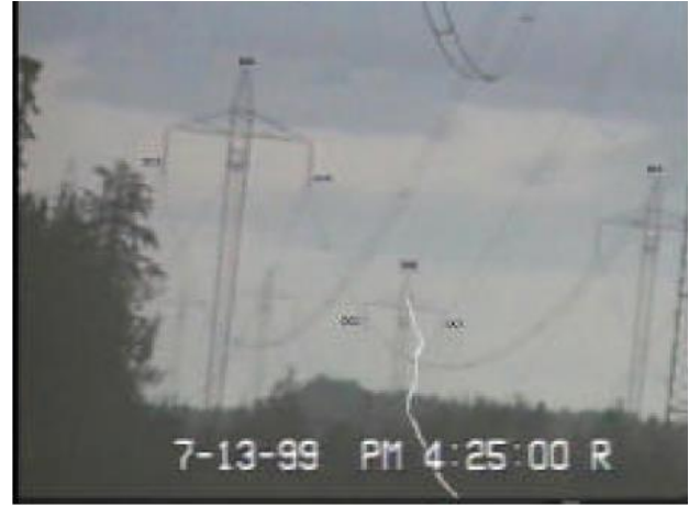
Figure 4: HVDC flashover captured on video [2].
