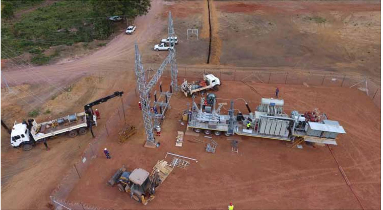
*The Zest Energy mobile substation in position on site, connected to the SNEL electrical network. The photograph shows preparations for hot commissioning and energising in progress.*
