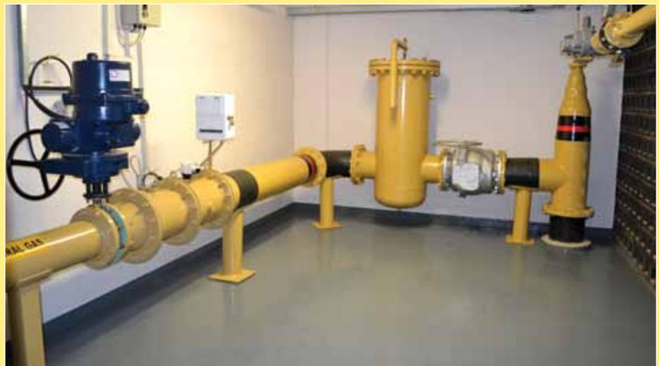
Incoming gas is at very low pressure, which makes it an extremely safe transporting mechanism. The main gas valve is held open against a spring and will shut-off automatically as soon as any sensor detects a leak.
