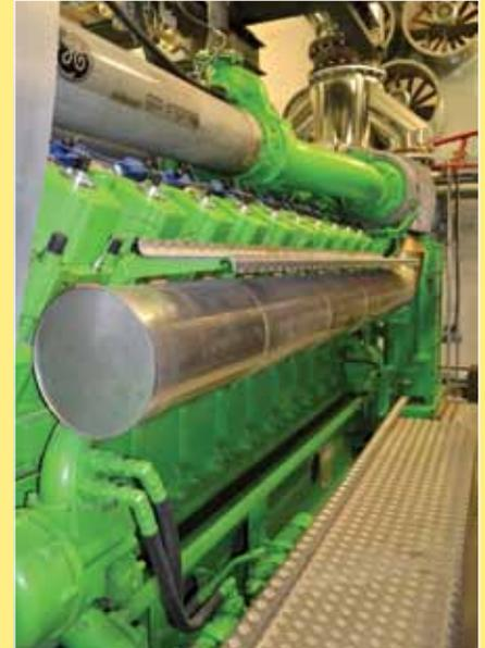
One of the four J 620s from GE installed at the Absa energy centre in Johannesburg. These 20 cylinder reciprocating gas engines have a peak generation capacity of 2,8MW each and emit 40% less greenhouse gases than coal-based generation, making them one of the cleanest combustion based technologies available.
