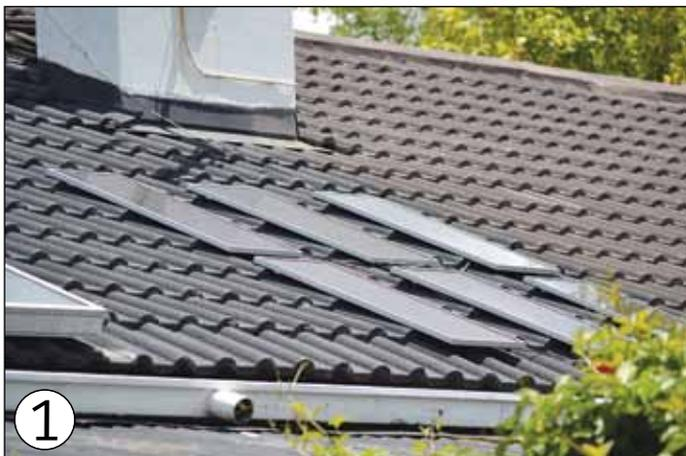
Six 10 W amorphous panels connected in parallel to give a theoretical 480 Wh from eight hours of sunshine. Actual power output of around 270 Wh was achieved, calculated based on recharging the battery after three hours of use.
