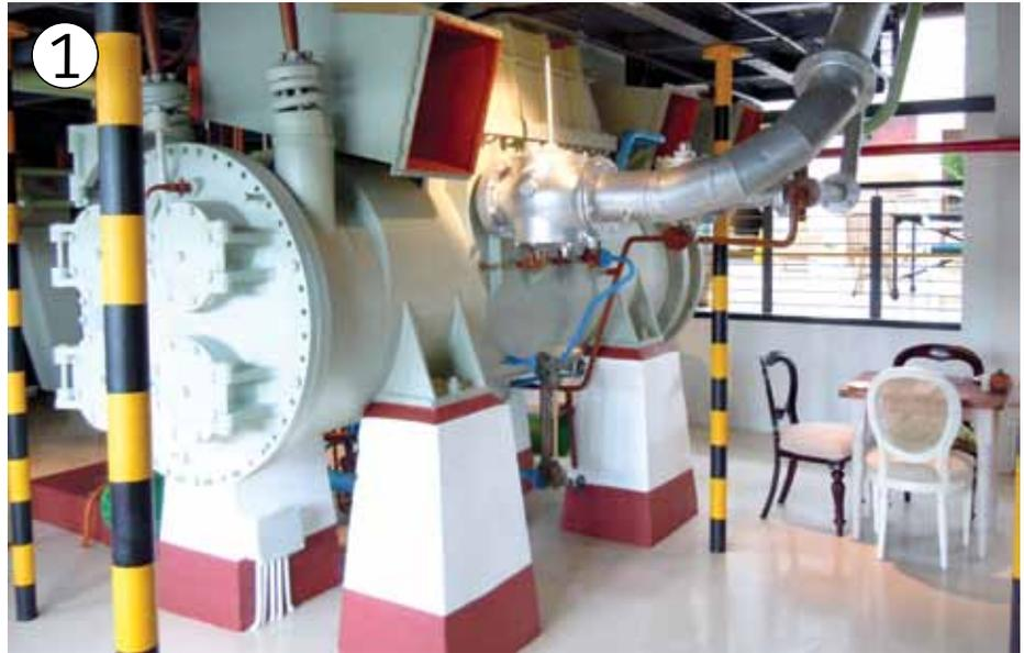
control panels that were retained in position over three levels! The generating plant consists of five turbine generators, with a combined total supply of about 10MW. The largest unit is rated at 2500kVA, while three tandem generators are rated at 1875kVA each. These three are thought to have been assembled in Grahamstown in 1923, before being purchased by Thesens in the 1940s.
