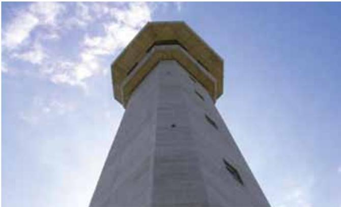
The 40 m concrete radar tower from below.
