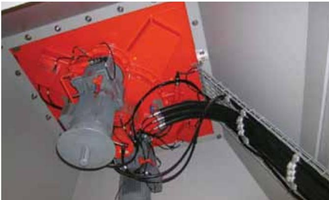
Antenna motor, gearbox, RF and power cables.
