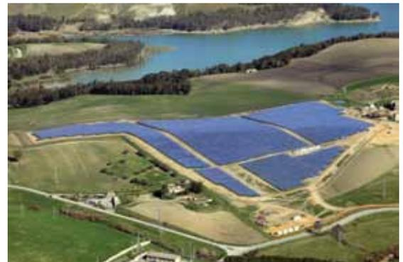
The 3,6MWp Sapeu fixed tilt PV installation installed in Sicily, Italy as a turnkey project by ABB in consortium with the panel manufacturer.
