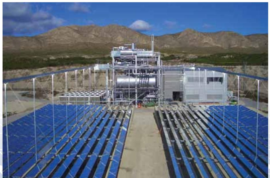
Novatec Solar's Puerto Errado 2 Thermosolar Power Plant in Spain, a 30MW linear Fresnel CSP plant due for completion 2012.
