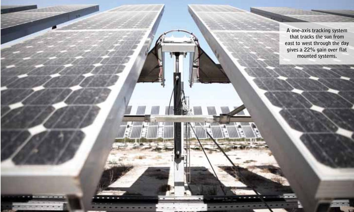
A one-axis tracking system that tracks the sun from east to west through the day gives a 22% gain over flat mounted systems.
