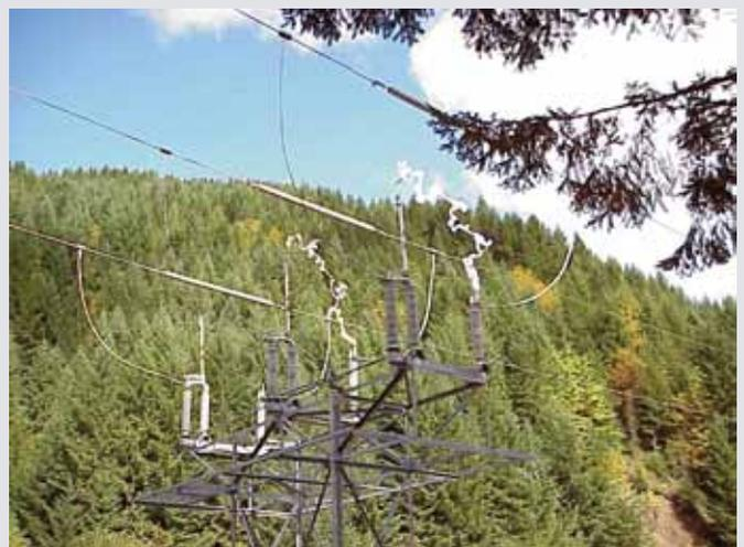
The picture shows what happens when a disconnect switch fails open properly. This was a 115 kV quick break disconnect that had exceeded its switching capability while attempting to de-energize a 40 km section of transmission line Tillamook, Oregon. At times the disconnect switch operated properly, but not this day. As can be seen, one phase successfully disconnected, but the other two phases did not. Luckily the operator was able to reclose the disconnect before it relayed out.
