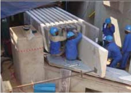
Figure 4: 360,000 Amp DC positive aluminium Busbar installation.
