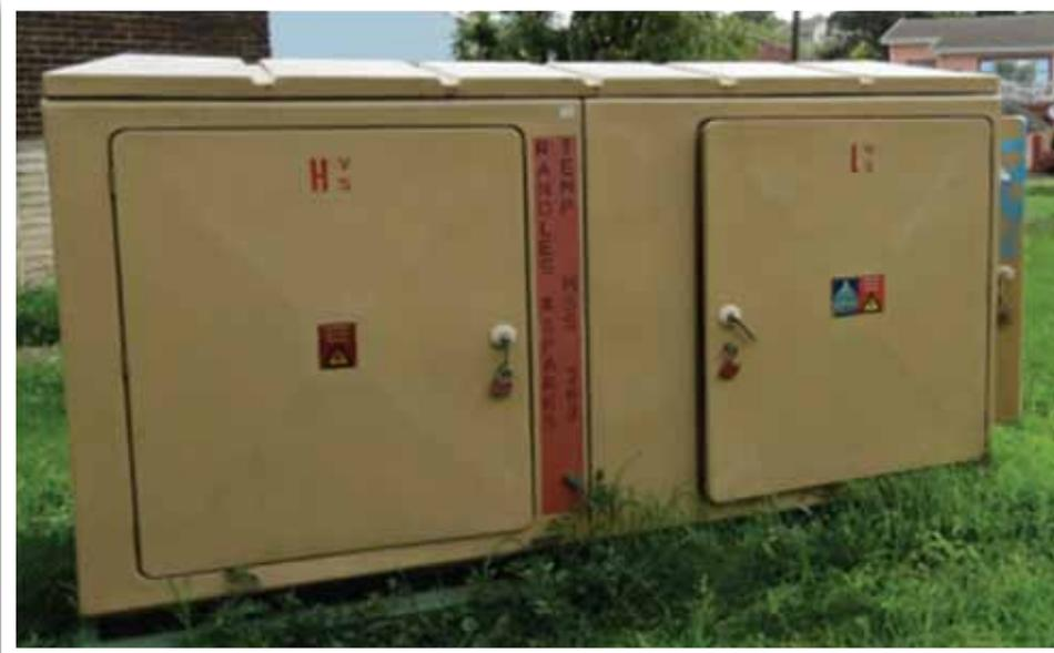
*Figure 1: Minisubstation containing 11kV/400V transformer, 11kV ring main unit and low voltage circuit fuses*
