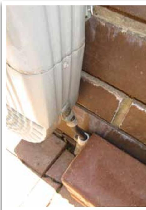
Figure 1: Example of earth bonding at SAIEE House.
