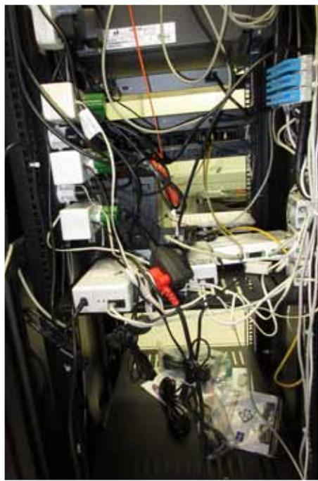
Figure 3: Showing unacceptable rack wiring.
