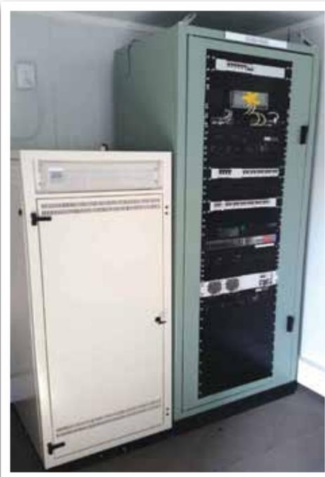
*Figure 4. Battery Back Up and Communications Panel*
