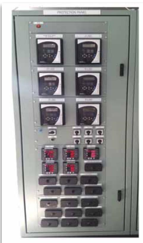
Figure 2. Control Room Metering and Protection Cabinet
