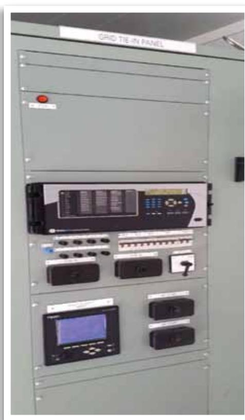
Figure 3. Control Room Grid Protection Panel
