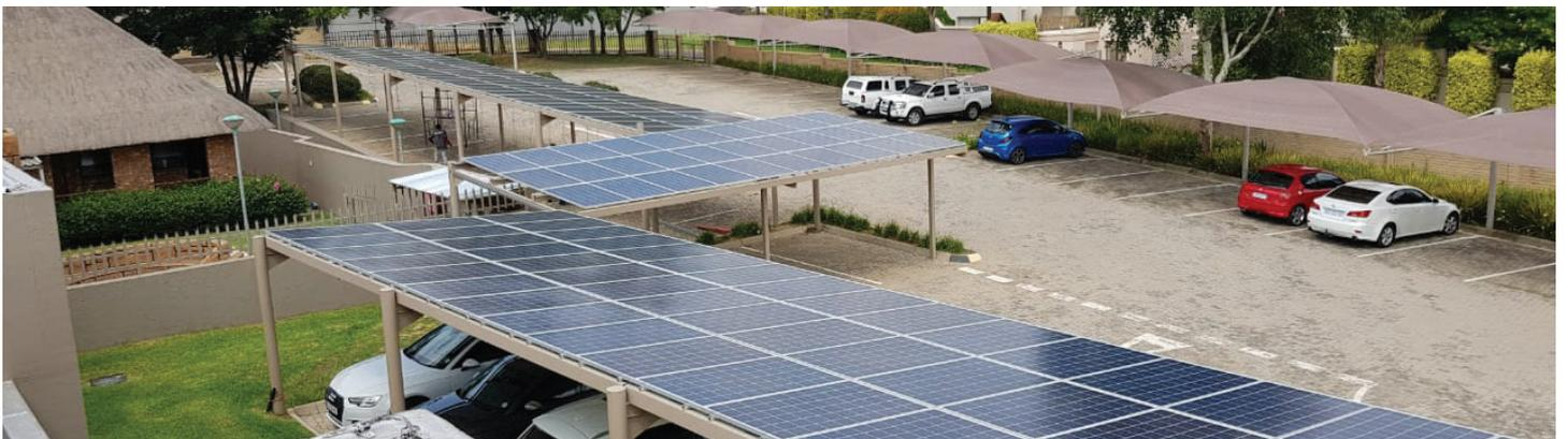
Hanonox has recently completed a 182kWp grid-tied solar project for financial services provider, MHA Management Holdings in Johannesburg. Hanonox's technical and design teams undertook the entire project scope - from modifying the existing carport structure to allow for panel mounting, to installing and commissioning the system in January 2019.
