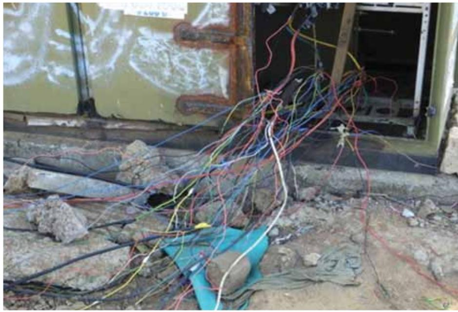
Figure 2: Typical illegal connection from mini-sub.
