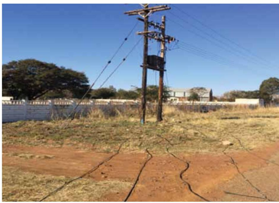
Figure 3: Typical illegal connection from Dx Transformer.
