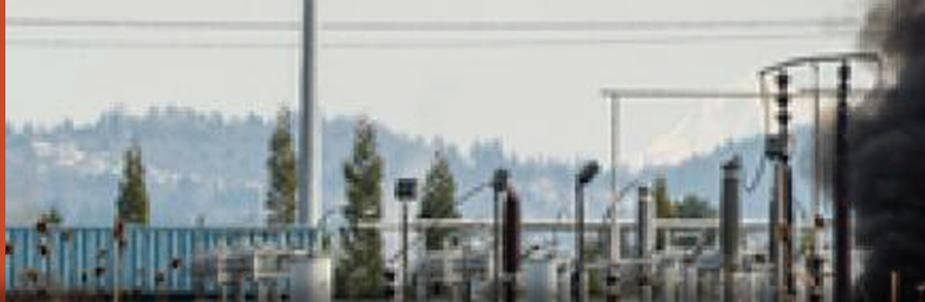
high temperatures. As the arc expands, so does the volume of these gasses and the transformer tank will eventually explode due to static pressure increase inside the tank caused by pressure waves travelling inside the transformer tank.
