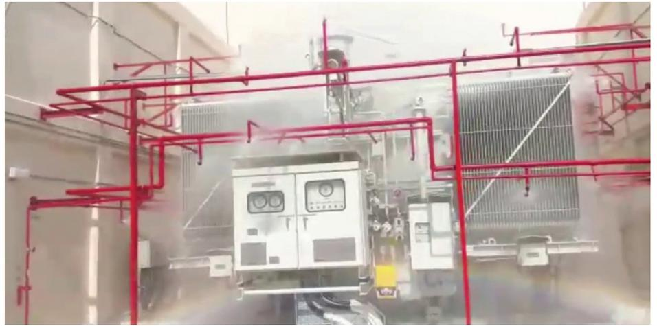
Figure 1: Transformer Sprinkler System
