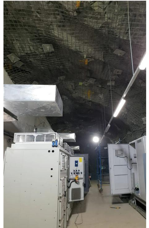
*The WEG MVW3000 VSD installed underground at a gold mine in Ghana.*
