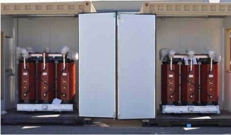
*The Trafo dry-type transformer is ideally suited to this application as it can be mounted inside the modular structure.*
