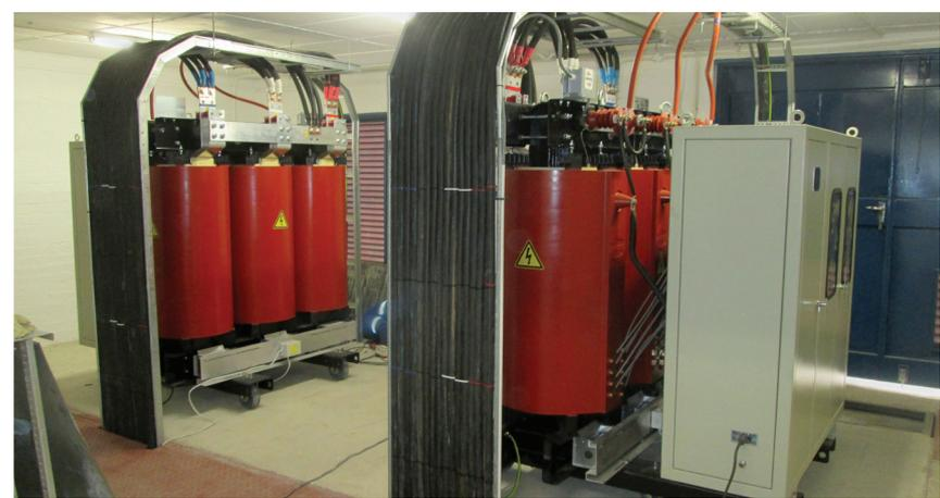
Two 1250 kVA 11 kV/400 V dry-type transformers with complete with on-load tap changers.
