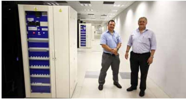
William Blackbeard (left) and Neil van Blerk in one of Vodacom's new Data Centre halls, which are illuminated by recessed high performance T5 light fittings, controlled by individually fitted passive infrared occupancy sensors.
