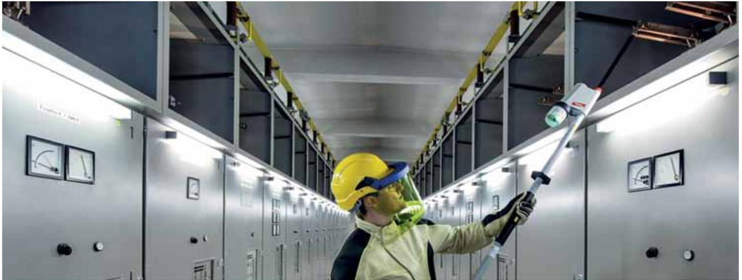
DEHN Africa has introduced the new PHE4 series of voltage detectors to improve safety during maintenance of electrical systems and installations. The detectors provide reliable information in all weather conditions – wet and dry – and can be used both indoors and outdoors.
