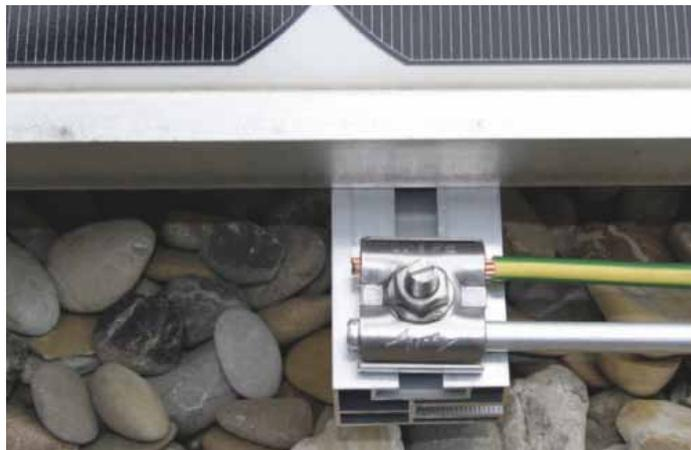
Figure 3 - UNI earthing clamp: A stainless steel intermediate element prevents contact corrosion, thus establishing reliable longterm connections between different conductor materials.
