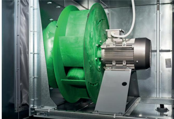
*Motor-fan machine set. Over 50% of motor failures are due to premature bearing failures. Many of the rotating machine faults that can be diagnosed with vibration condition monitoring such as unbalance, misalignment, and mechanical looseness, directly impact the motor's bearings*
