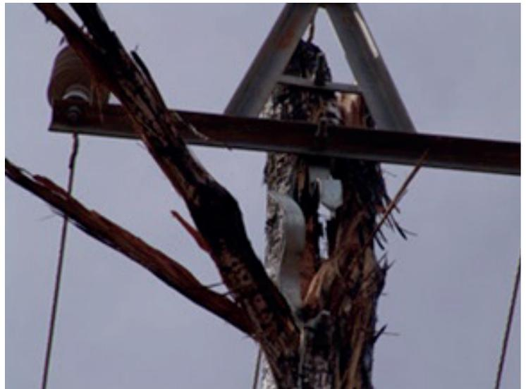
Figure 2 : Example of pole damage in the wood gap [1] (above left), mitigation solution [9] (above right) and a rare case of damage to a pole in the wood gap with spark gap inserted [9] (below)
