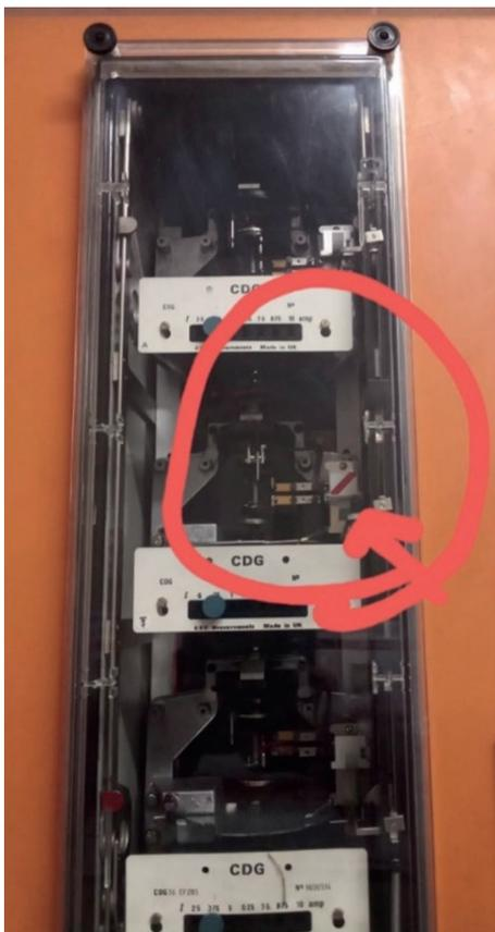
Fig. 9: Operated Protection Relay (Earth Fault Flagged)
