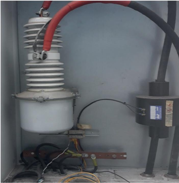
Fig. 4: The VersaVac Breaker and the Neutral CT
