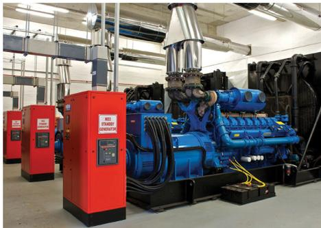
Six 2 000 kVA open type synchronising generator sets
