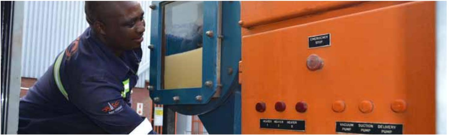
When drawing the oil sample, the sampling technician will also do a visual external inspection of the transformer against a checklist as this will pick up any physical issues with the transformer. Evidence of leaks or a change in colour of the silica gel will be a clear indication that there is moisture ingress. The general condition will also give an indication of corrosion.
