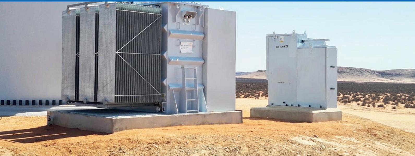
*One of the padmount 2.7MVA 0.69/33kV inverter transformers produced for the wind turbines of the Kangnas wind farm in the Northern Cape in Round 4.5 of the national REIPPPP programme*
