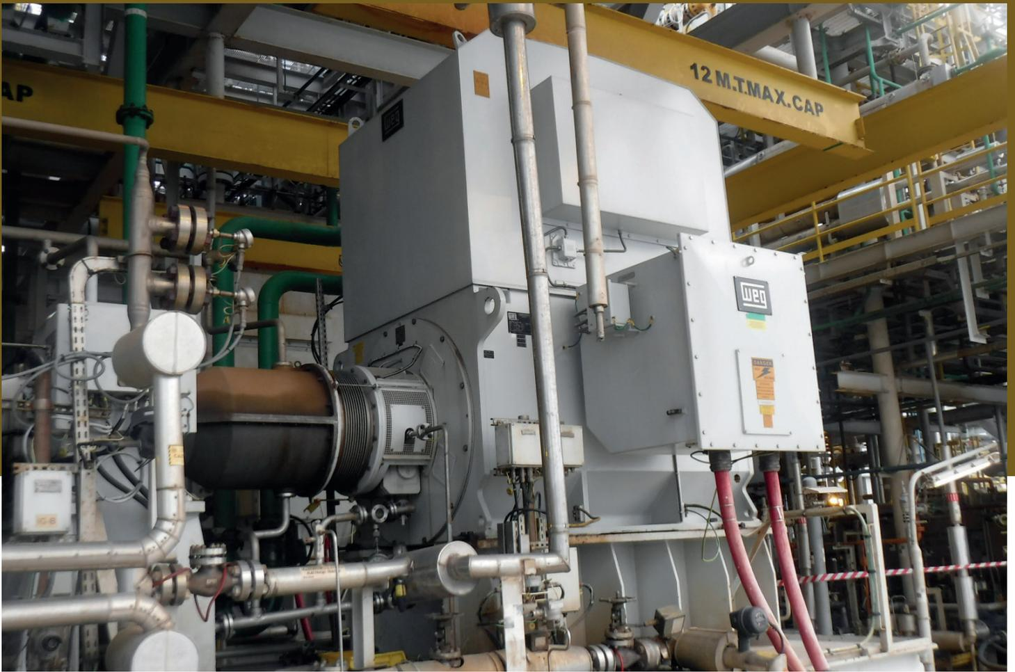
*The coupling between the WEG motor and the compressor.*
