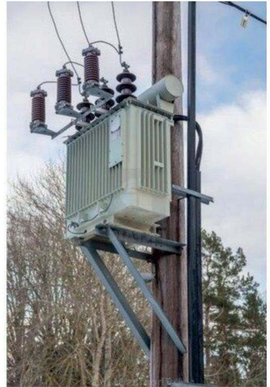
Figure 1: In a medium-voltage transformer installation, there are typically three primary earthing systems.
