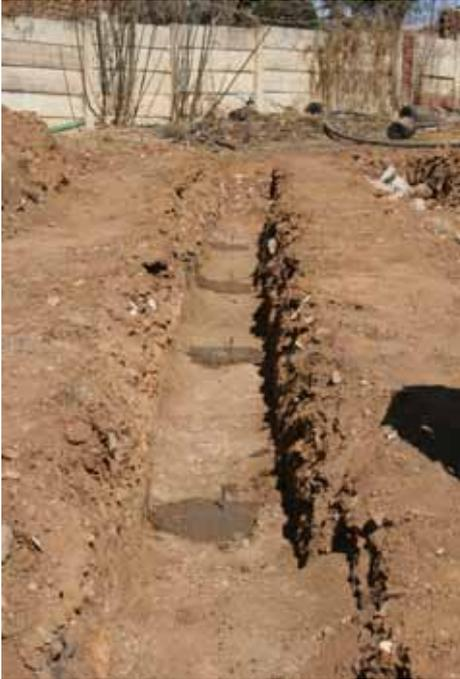
1. The trench with the anchors cemented into the bottom of the trench. This was done the previous Wednesday, to allow the cement to set for 2 days.
