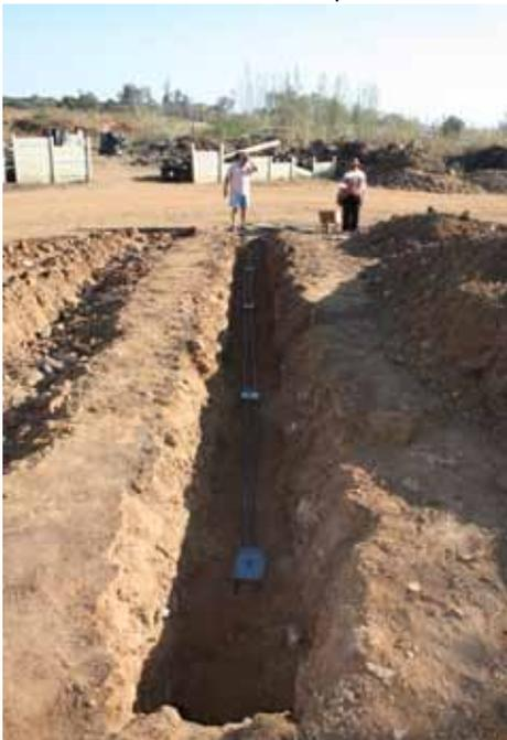
2. The cable was installed and secured with the 4 securing plates. The front of each of the devices, with the cable in the front, were sprayed with silver paint, to show any possible slip that occurred.
