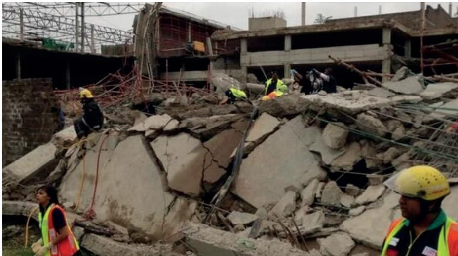
**Figure 4:** Collapse of Tongaat Mall during construction
